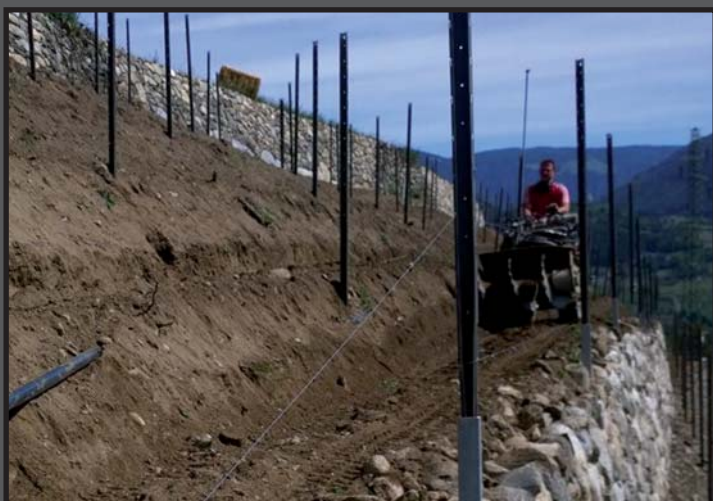
SERVICE SPECIALIZED WORKS
